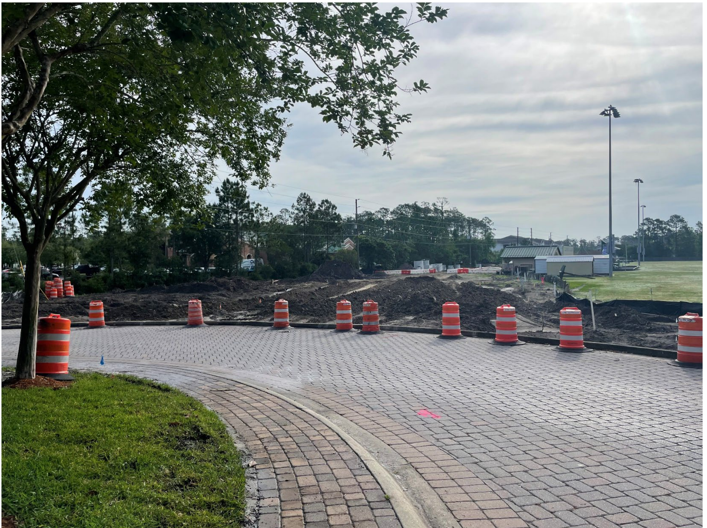
Radar Road (looking east from Town Center Boulevard round-a-bout)
