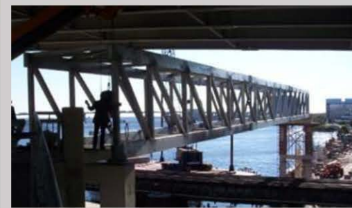
Threading the needle: placing pedestrian bridge over FEC rail, & under the Acosta, on top of support structure.
