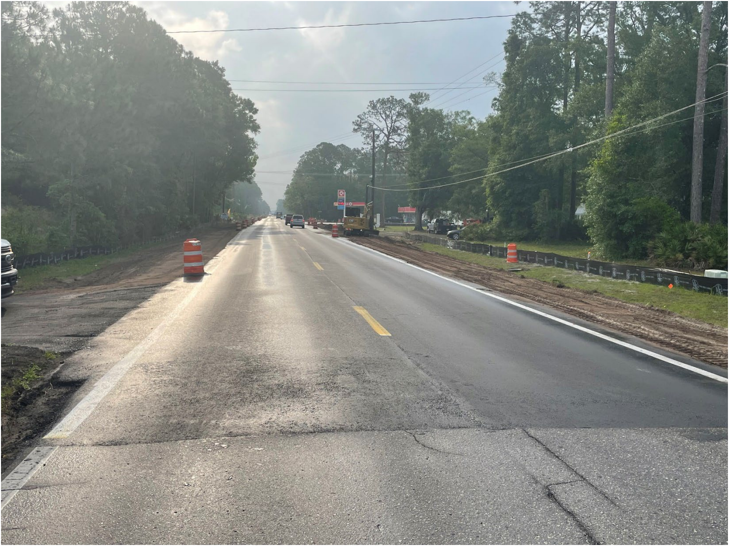
Old Jennings Road (looking east)
